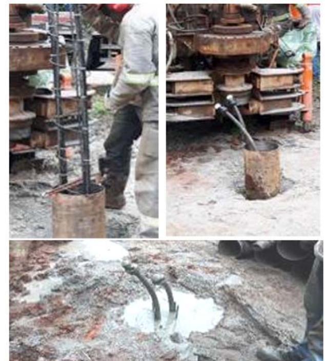
Fig.4. Construction of the energy pile: installation of the reinforcement cage with a U-shaped heat exchanger tube
