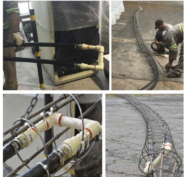
Fig.3. Installation of the U-shaped exchanger tubes in the reinforcement cage of the micropile
