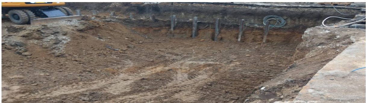
Fig. 2. Leveling of the piles.
