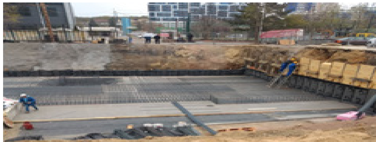
Fig. 3. Execution of the trench cladding.
