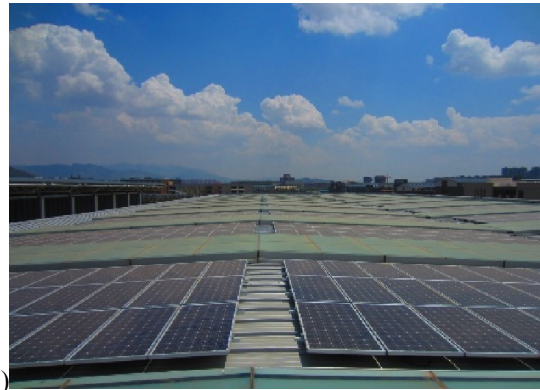
Fig.1. Yunnan Normal University rooftop PV systems. (a) The 256.50kWp installation capacity on the roof of the library, (b) The 90 kWp installation capacity on the roof of the indoor swimming pool, (c) The 652kWp installation capacity on the roof of the sports training centre
