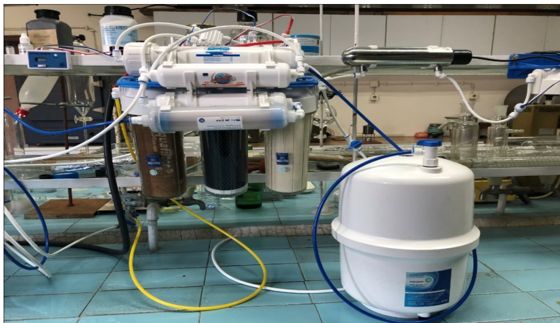
Fig. 2. 7 - stage reverse osmosis system with UV – disinfection (Module 1).
