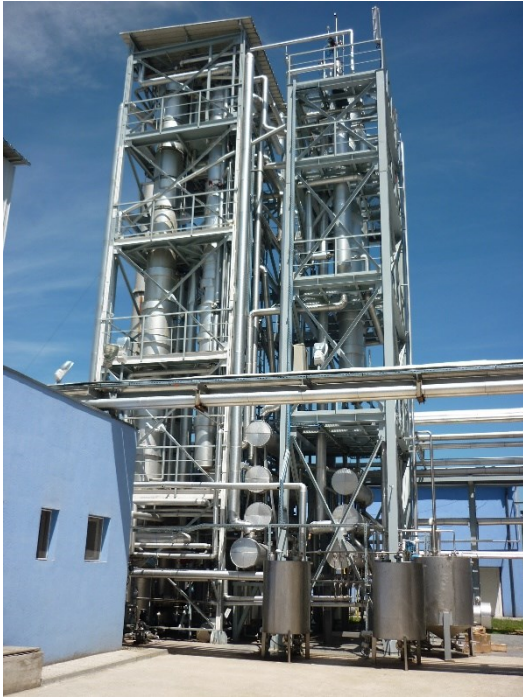
Fig. 17. Photograph of a rectification plant for ethanol production with productivity of 20000 litres/24h consisting of five columns with Holpack packing
